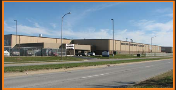
MECO OMAHA's 200,000 sq. ft. facility on ten acres of land in Omaha, Nebraska.
